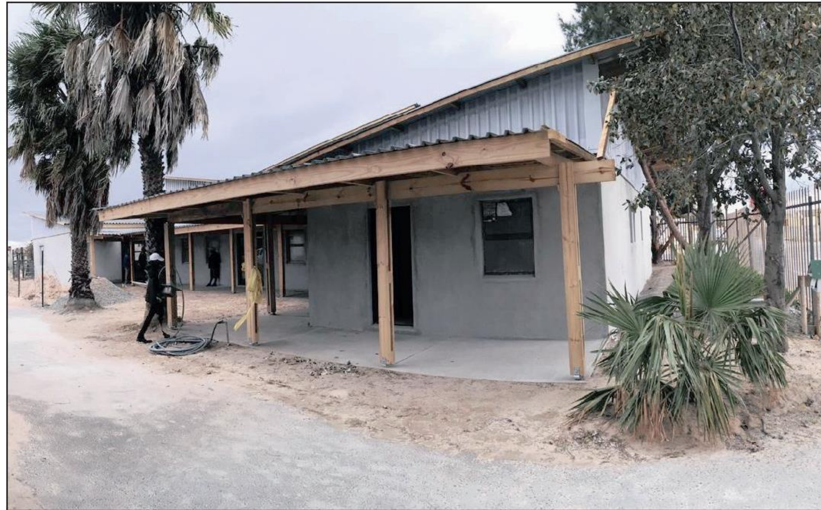
The new buildings at Noluthando day care centre in Khayelitsha were built using Selcrete blocks.
